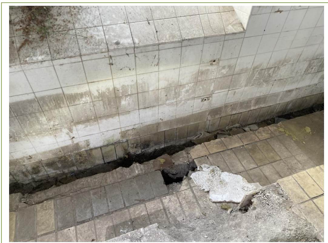
Ceramic floor tiles in building 5
