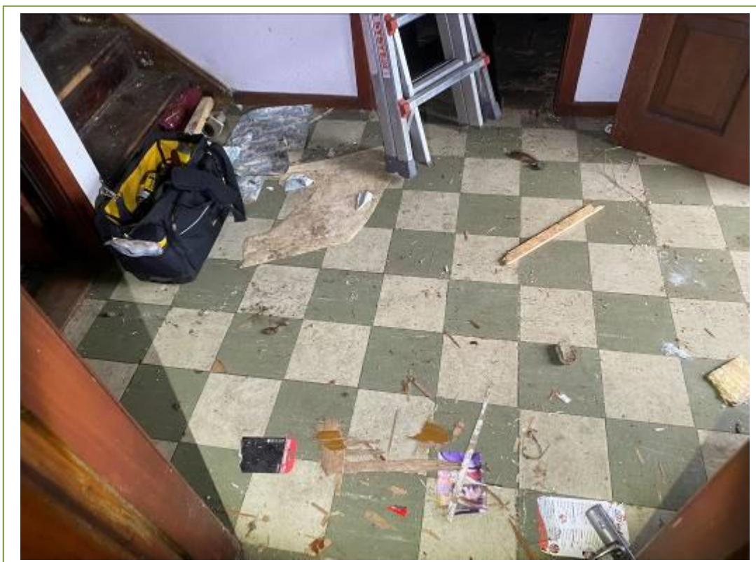
Floor tiles sampled from the hallway
