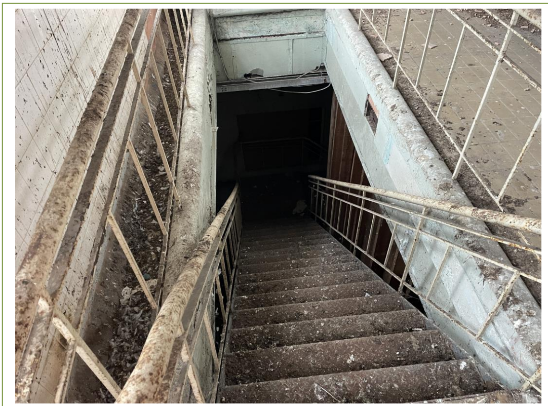
Asbestos insulation board on the walls of the stairs to the 1 st floor in Building 12
