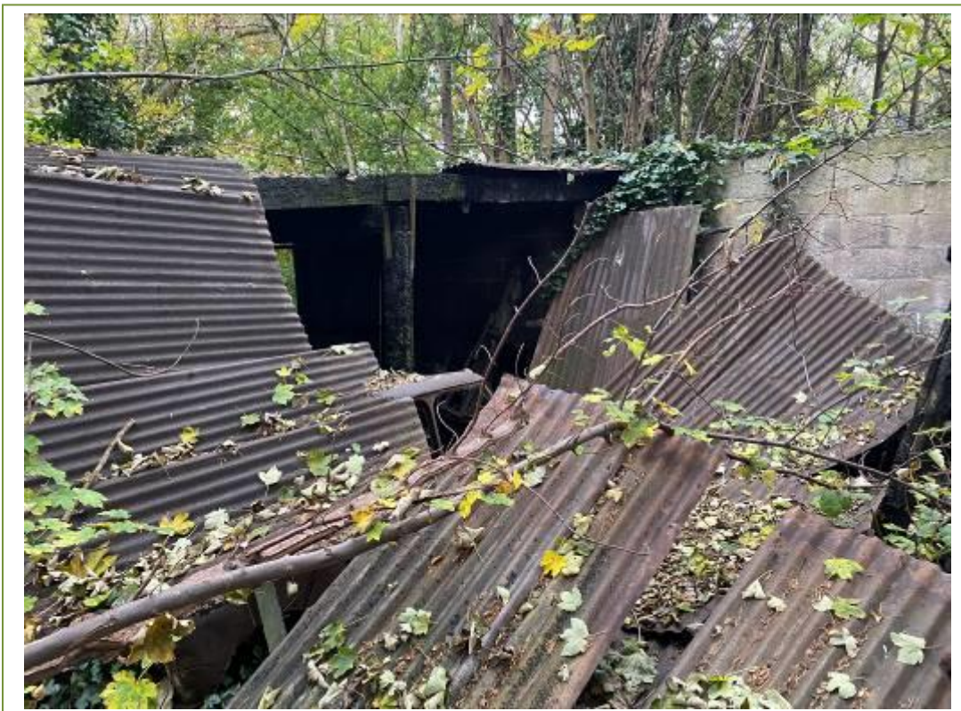
Metal cladding on the rear outbuilding
