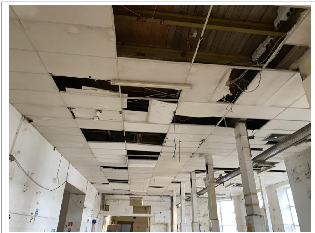
Plasterboard ceiling tiles in building 5
