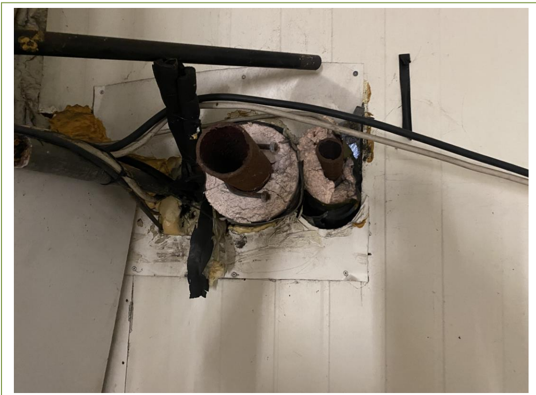
Pipework insulation sampled in building 5
